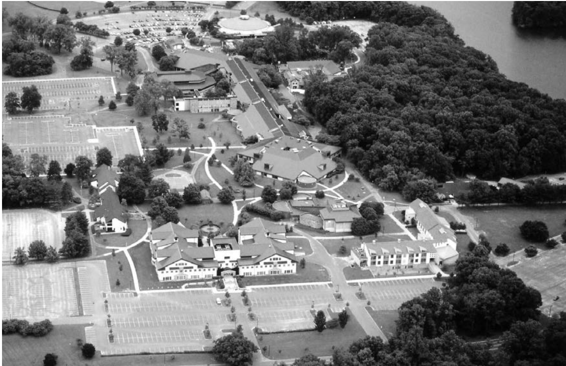
Aerial view of a portion of Brookdale Community College as it stands today (2005). Converted barns are now less recognizable as the stables they once were. The Center for the Visual Arts building in the bottom right of this photo is partially formed by one of the old barns.
