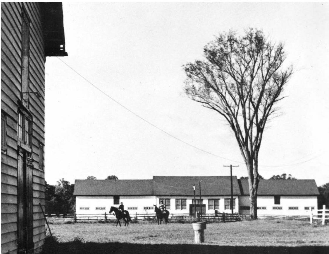
The horses being ridden out of the barns so that renovation can begin.
